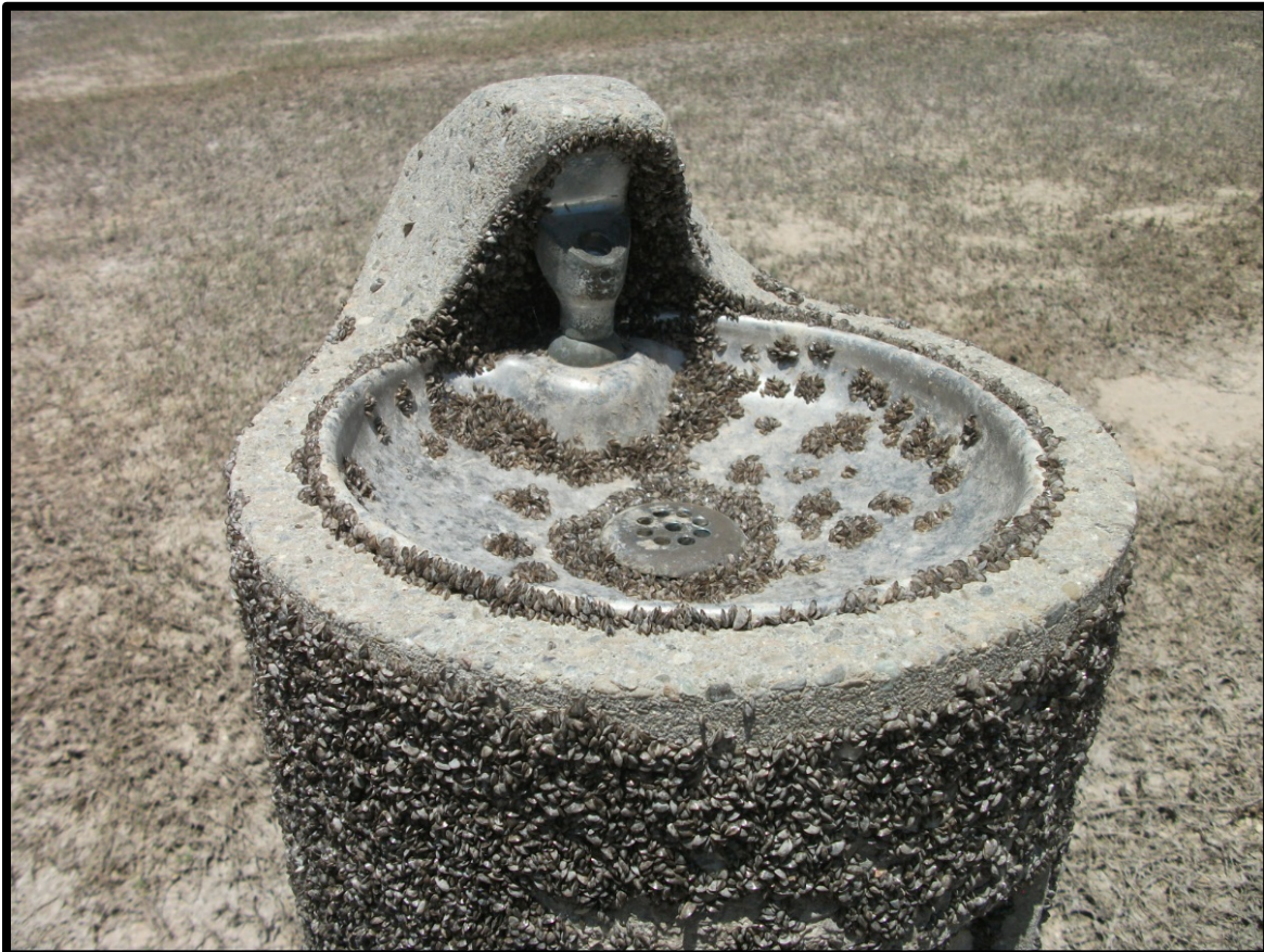
Photo 6.2 Concrete Drinking Fountain Inundated for 45 days. (USACE Photo)
